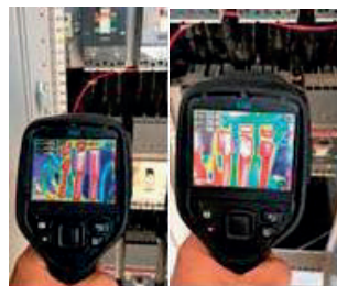
Figure 10. Inspection of inverter with thermal camera
