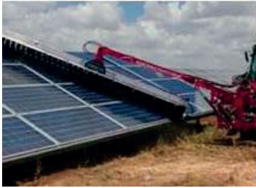
Figure 7. Panel cleaning with cleaning machine
