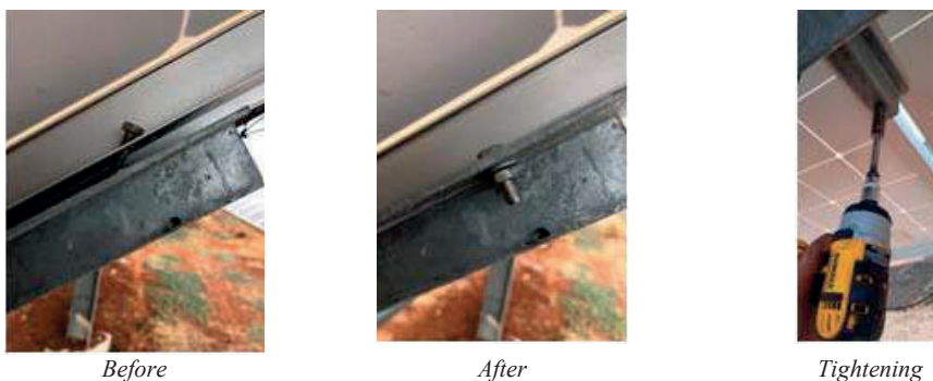
Figure 11. Checking the bolt connection and fixing it.
