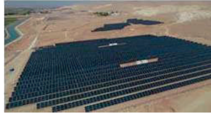
Figure 5. Fixed-tilt solar PV plant
